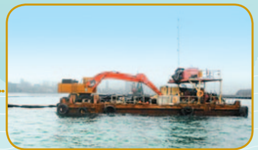
疏浚工程前安裝隔泥幕 Installation of silt curtain before dredging
